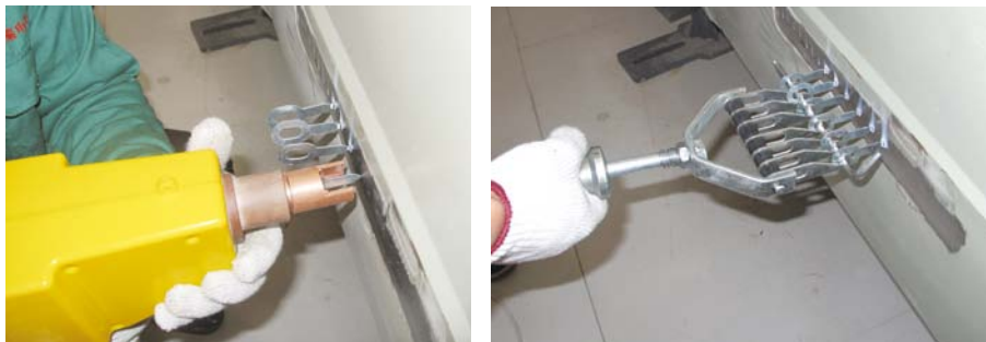
Twist pads welding and pulling
